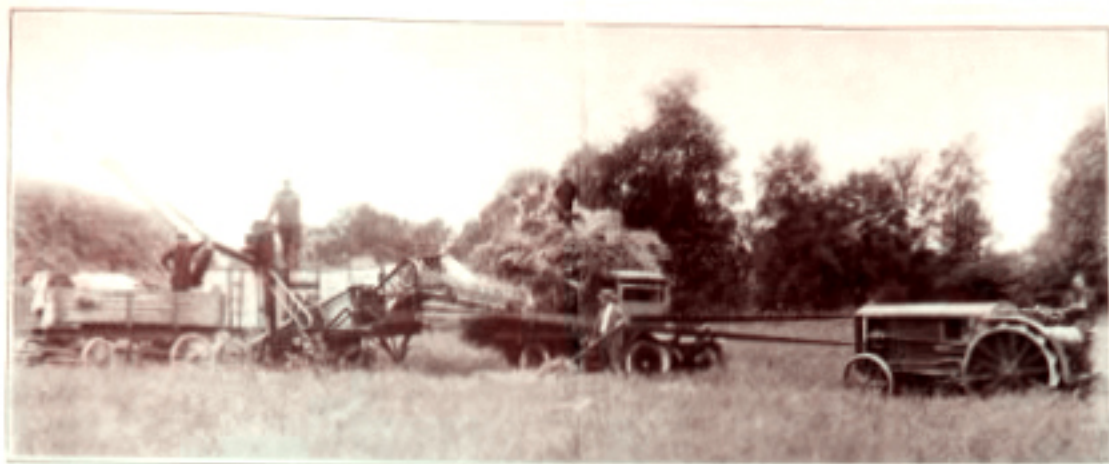
Bryan Light Steam Tractor and Truck Operating a Threshing Outfit.
